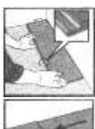
STEP 1: Start in the left hand corner of the room with the tongue facing into the room. For uneven walls you may need to scribe the profile onto the first row and cut accordingly. Take care to ensure a minimum 14mm expansion distance to walls using spacers or wedges.
